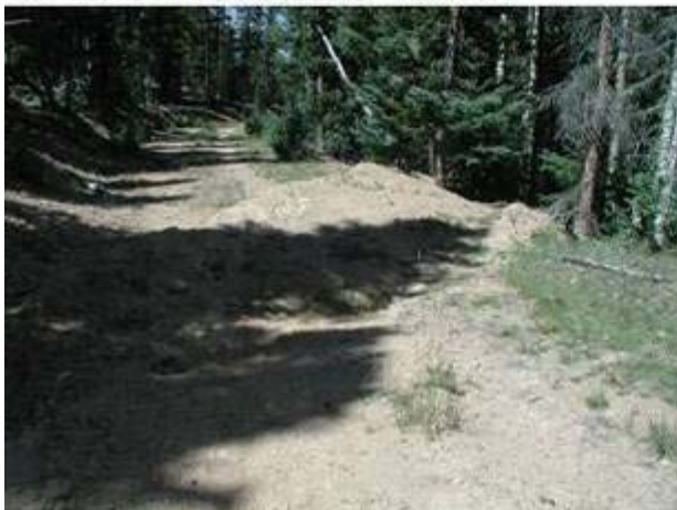
HPP #36 UTM 475353/4076437 water bar
