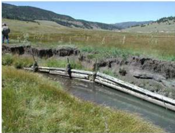
HPP#80 bank erosions stabilization structure
