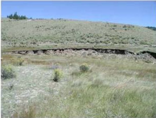
HPP#73 UTM 479276/4070451 Bank erosion on Comanche Creek
