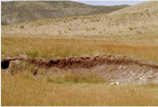
HPP#65-66 Left fork of the north fork of La Belle: #65 road cut, grass over but bottom showing gravel and soil movement, drops into drainage with major head cuts, #66 up hill from bottom of road.
