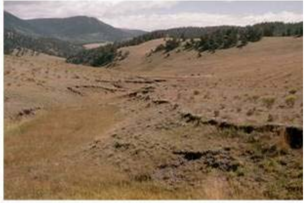
HPP#62 UTM 0473268/4068408 La Belle Lodge—earth dam in danger of breaching, cut lower than spillway—view NE 50 degrees
