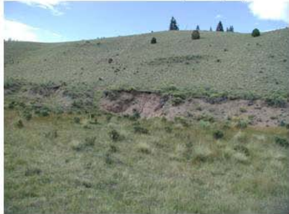
HPR#16 UTM 472636/4074110 Big eroding slope
