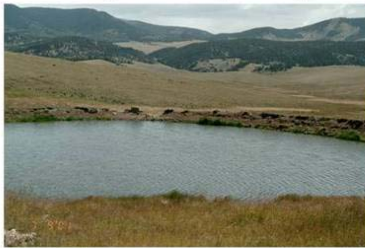
HPP#62 UTM 0473268/4068408 La Belle Lodge—earth dam in danger of breaching, cut lower than spillway—view NE 50 degrees
