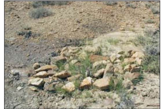
One-rock dam at Torreon Chapter, 2002, doing what one-rock dams are supposed to do, hold water and grow grass.
